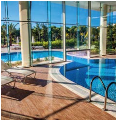
Swimming Pool Dehumidification Unit
